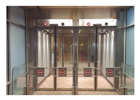
In November of 2015, Eugene Airport (OR) installed their exit lane breach technology as part of their terminal expansion project. Two (2) Twin Extended (two full height doors with half-height gates) models were installed by record-usa. The exit corridor was tested and approved as unmanned by their local Federal Security Director (FSD) in August of 2016.
